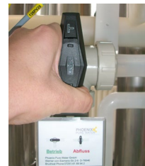
Three-way valve drain position
